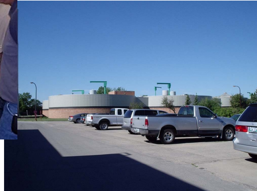
City Wastewater Treatment Plant, Winnipeg, Canada
