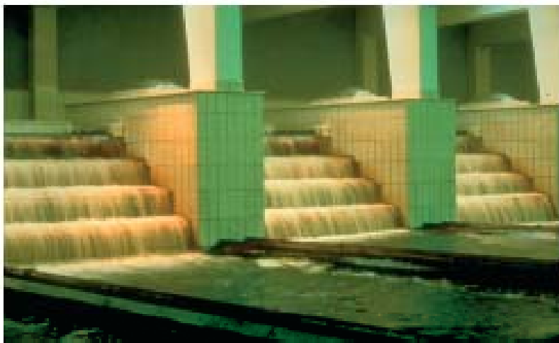
Figure 1 - Cascade aeration
